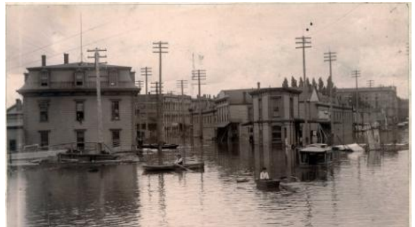
Flood of 1894 looking south on 1 st from Everett. Image: Norm Gholston.
