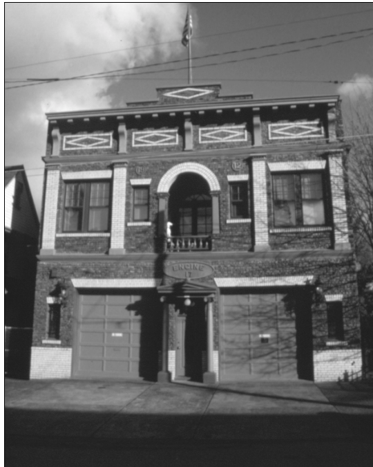
Portland Fire Station No. 17, 824 NW 24 th Avenue
