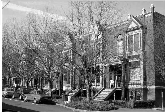
The Campbell Townhouses, 1705 - 1719 NW Irving Street
