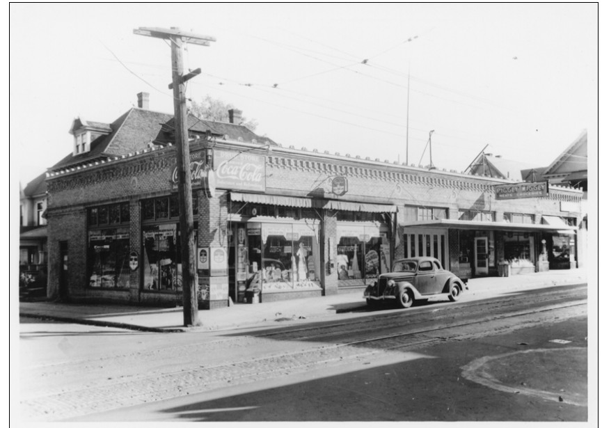
Looking southeast at 622 NW 23rd Avenue
